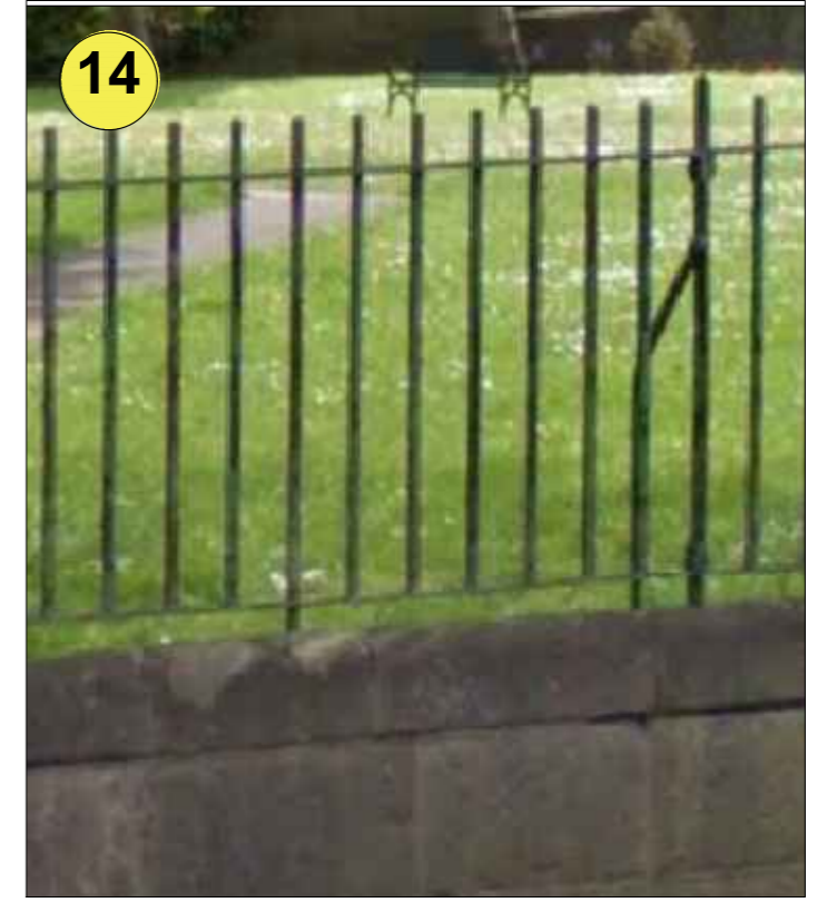
14 Existing Fence to be professionally Repainted, and wall repointed and repaired as necessary.
