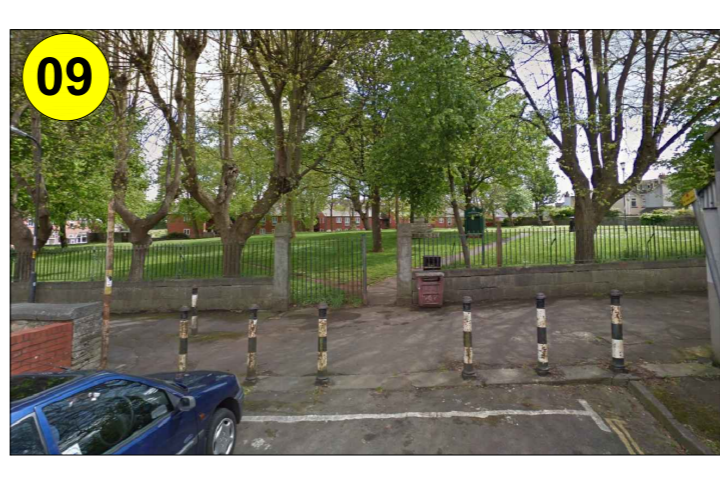
09 Bollards to be repainted.
