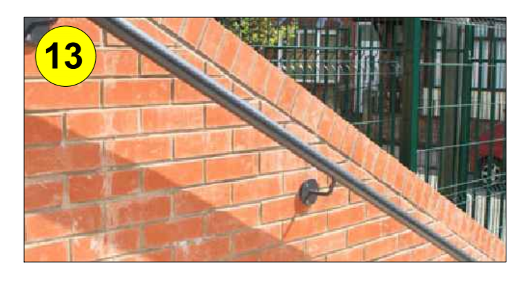
13 Provide and install new Stainless steel hand rail above existing steps.
